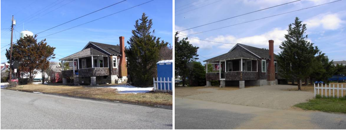
Figure 12.5 Elevating land and house. (a) Initial elevation of house in Brant Beach (New Jersey). (b) Structural beams placed under house, which is lifted approximately 1.5 meters by hydraulic jack in blue truck. (c) Three course of cinder blocks added then house set down onto the blocks. (d) Soil and gravel brought in to elevate land surface. (January through June 2005)
