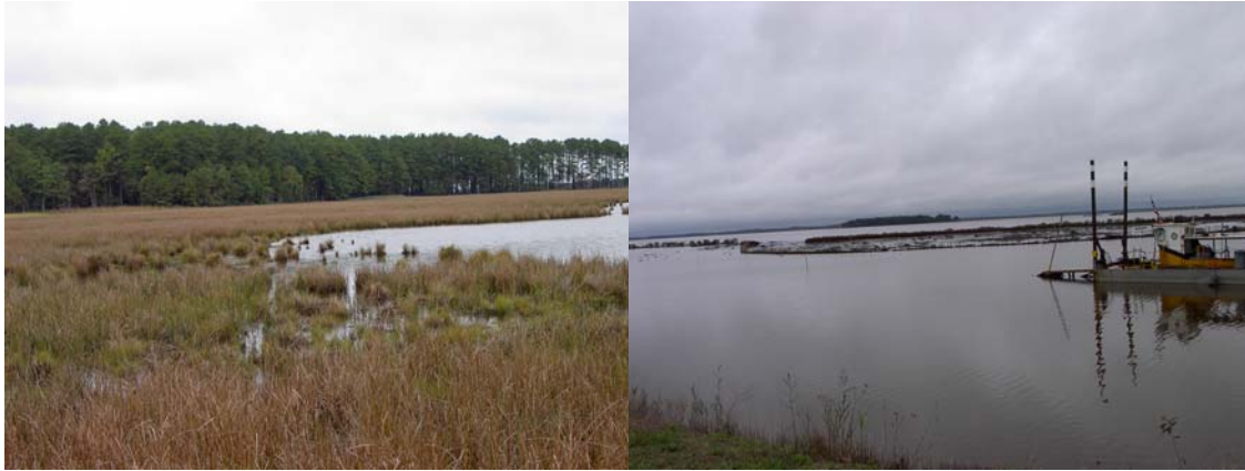
Figure 11.2 Responding to sea-level rise at Blackwater National Wildlife Refuge, Maryland (October 2002). (a) Marsh Deterioration. (b) Marsh Creation. The dredge fills the area between the stakes to create land at an elevation flooded by the tides, after which marsh grasses are planted
